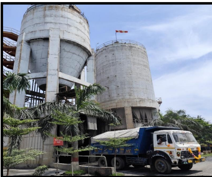
(Covered Fly Ash carrying truck)
