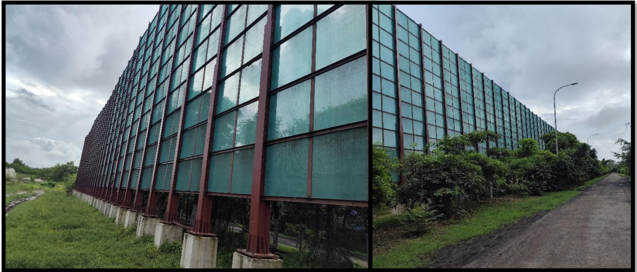
Metallic wind screen installed to control fugitive emission
